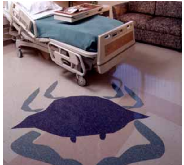
Every patient room in the Anne Arundel Medical Center's new Acute Care Pavilion has a multi-colored, custom-designed inset in the vinyl floor. Here, a crab was created using Imperial® Texture™ tile.
